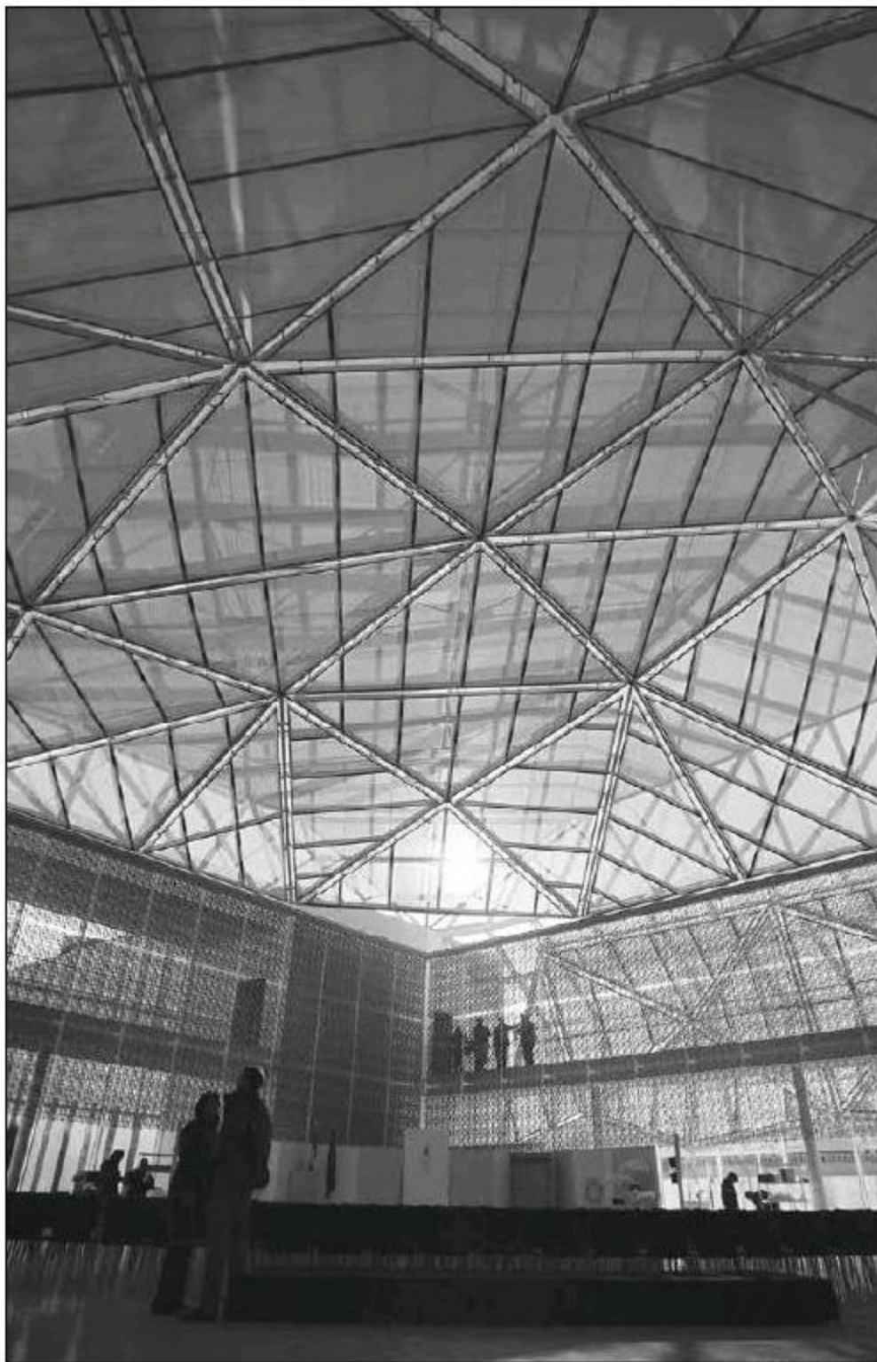
INTERIOR: A cast aluminum screen encloses the atrium. The pattern is a double layer of repeating hexagons and is inspired by Islamic design. Officials prepare for today's opening ceremony.
